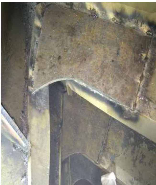
Renew brackets connection for SL 22.4 to SL 22.6, 12mmt 900 x 600 x 3pcs
