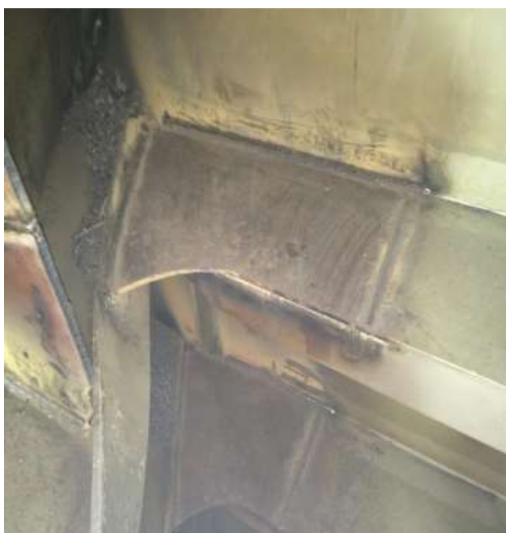
Renew brackets connection for SL 22.4 to SL 22.6, 12mmt 900 x 600 x 3pcs
