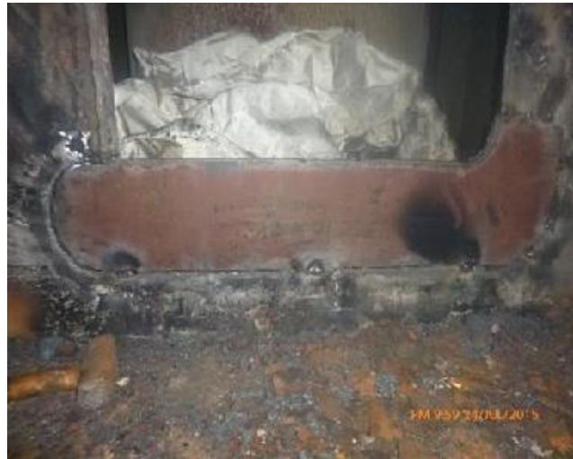
Replacement of 3rd door bottom part
