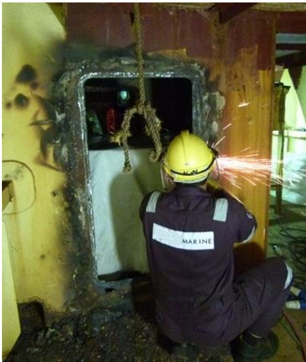
Grinding after cropping off
