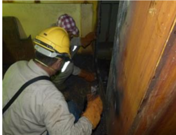
Replacement of 1st door bottom part
