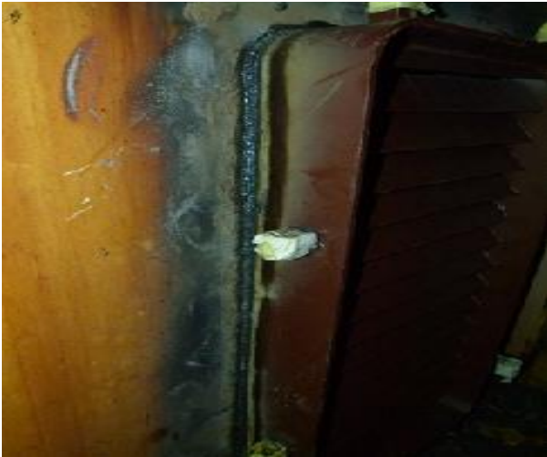
Full welding completed
