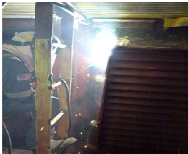
Fit up and commenced with full welding
