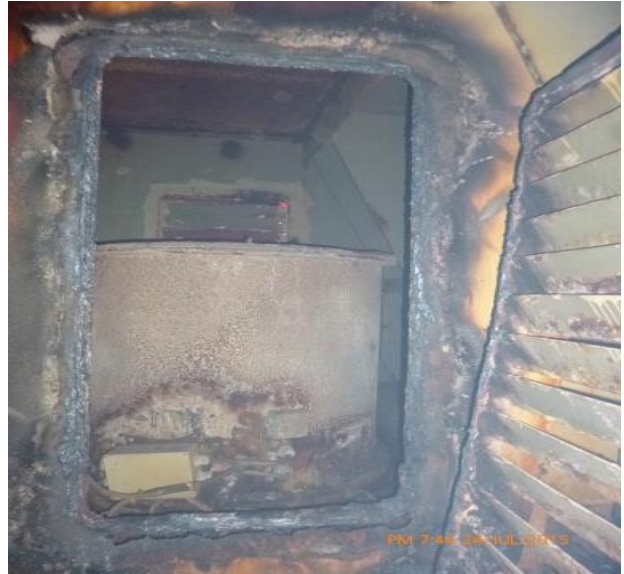
Ventilation door after completely crop off
