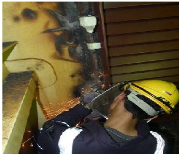
Grinding at the weldment
