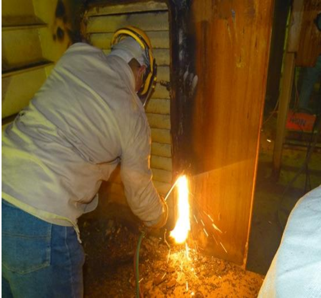
Cropped off all renewal door using flame cutter
