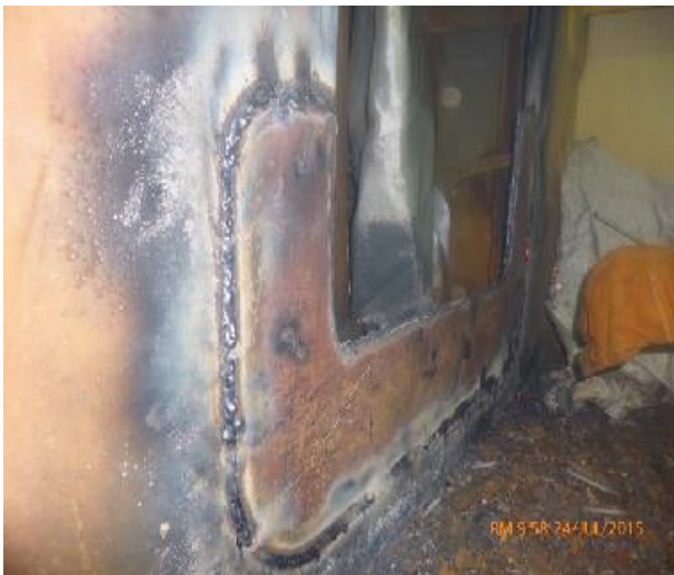
Replacement of 2nd door bottom part
