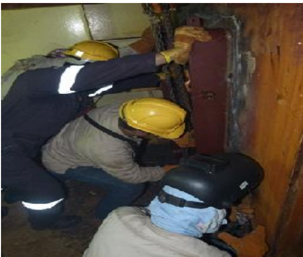
Hoist up new door using chain block for fitting
