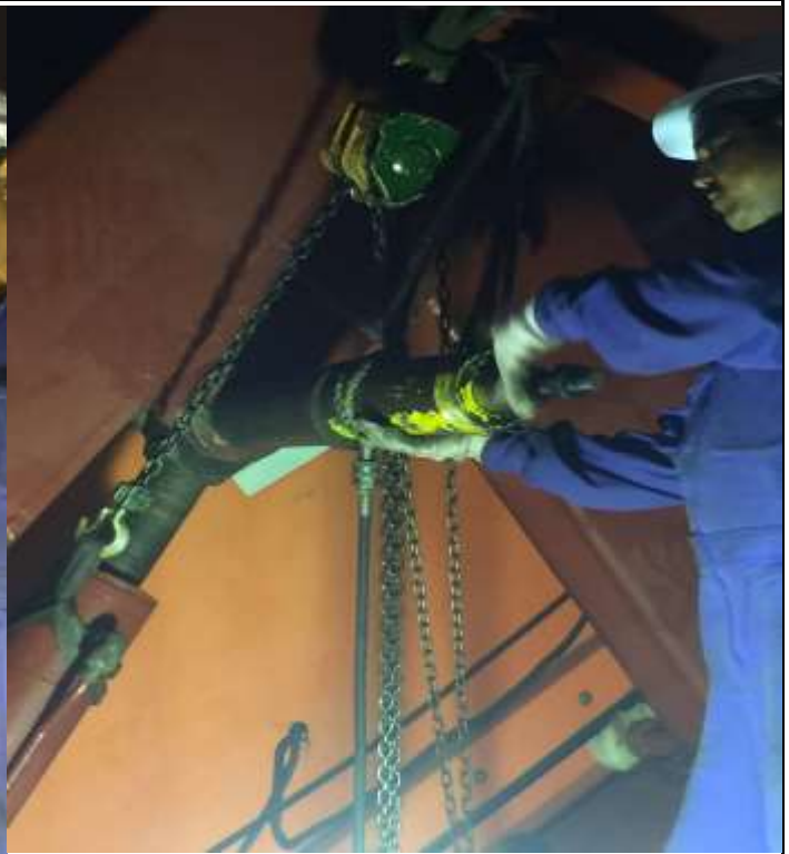
Hydraulic tools used to remove the pins with pressure after attempt to remove pin by hammering unsuccessful
