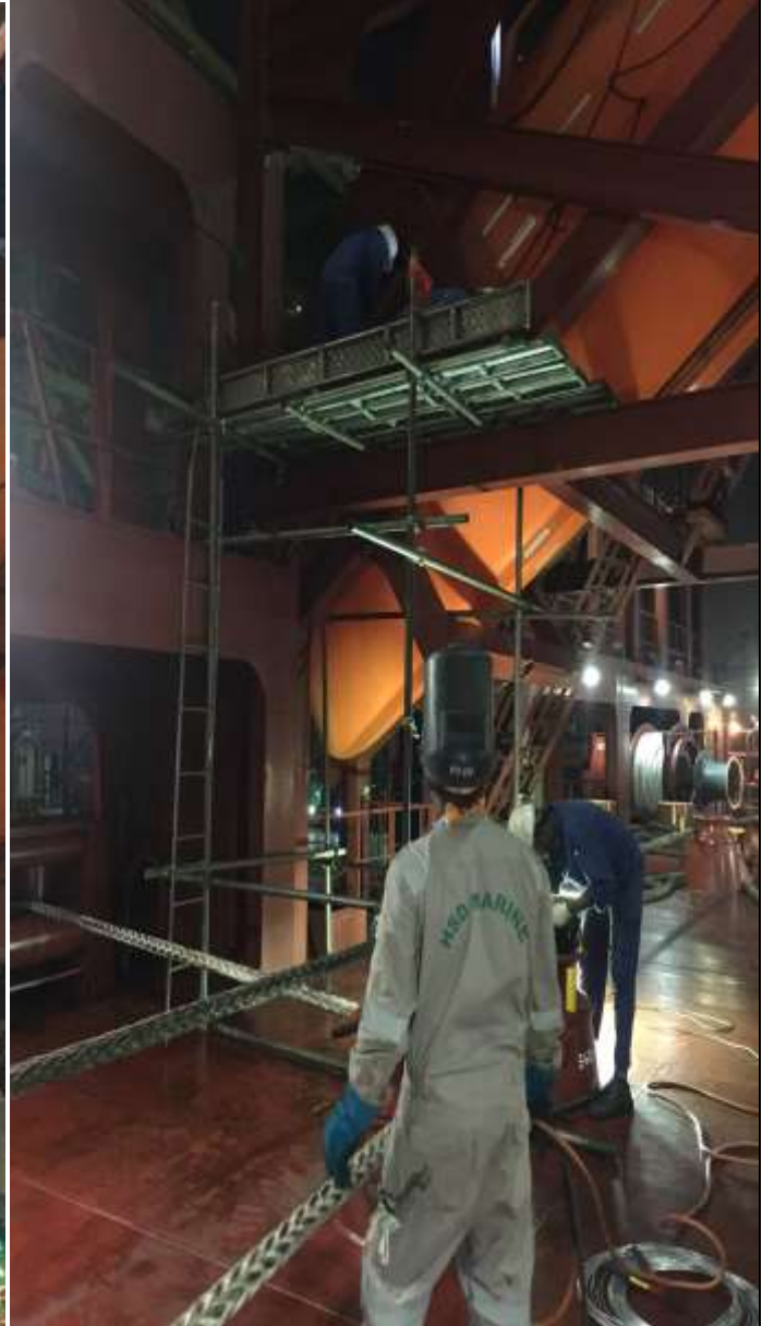
Erecting two tier staging to access hydraulic cylinder
