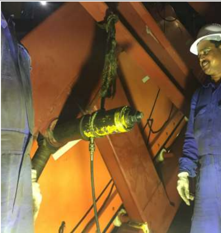
Hydraulic tools used to remove the pins with pressure after attempt to remove pin by hammering unsuccessful
