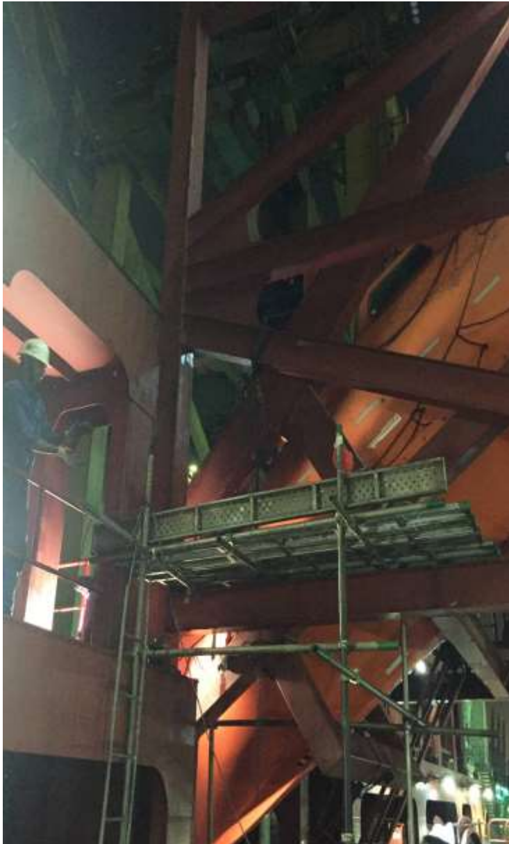
Erecting two tier staging to access hydraulic cylinder
