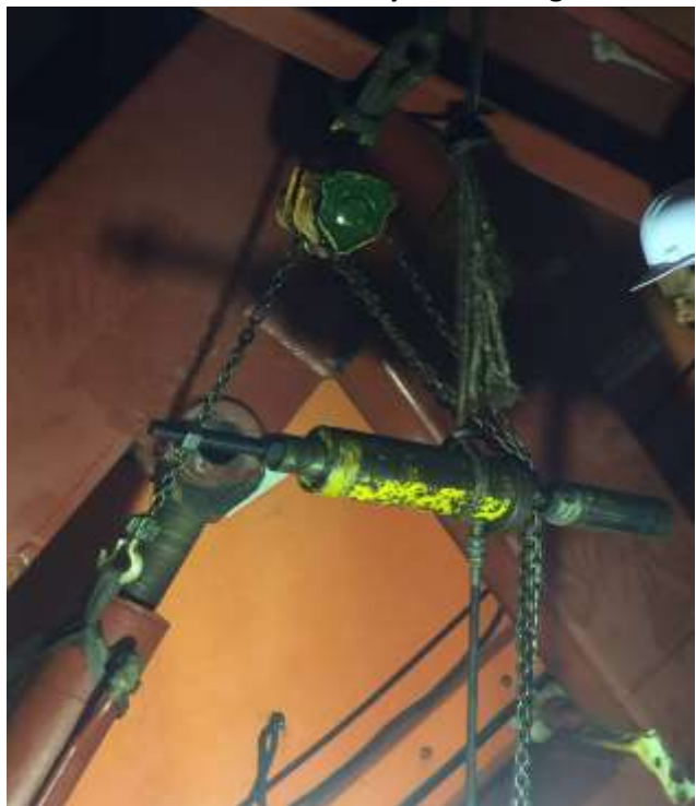
Hydraulic tools used to remove the pins with pressure after attempt to remove pin by hammering unsuccessful
