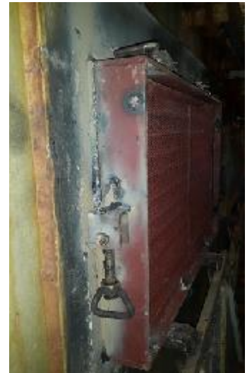
Installation of newly fabricated Louvers and fitting as well as alignment
