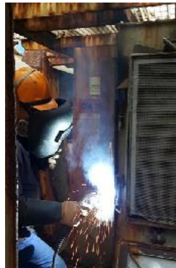
Installation of newly fabricated Louvers and fitting as well as alignment
