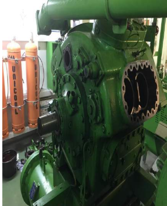
To remove the pulley, sleeve and seal for overhaul works
