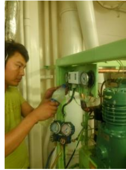
Carried out leakage test
