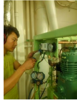
Carried out leakage test
