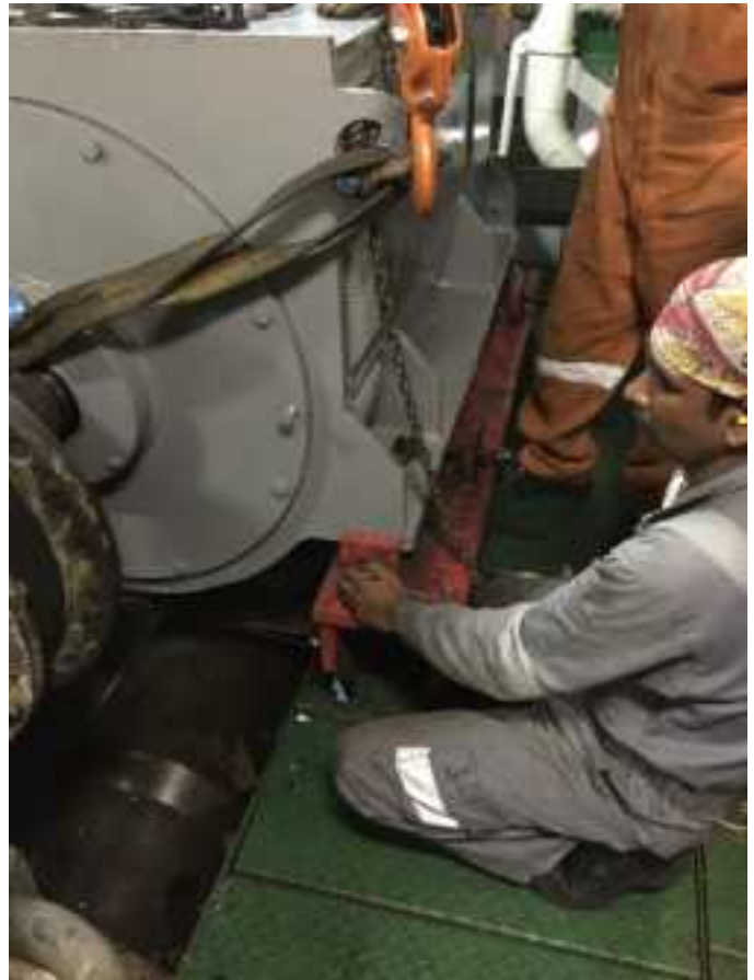
Adjusting alignment of generator & jacking bolts of foundation
