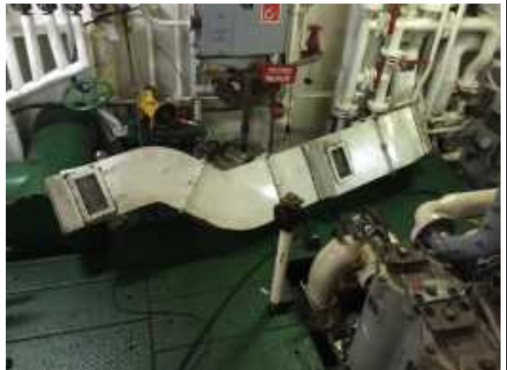
Removal of E/R air duct section
