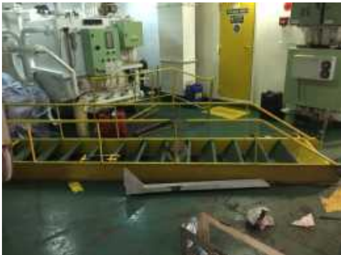
Removal of E/R access ladder
