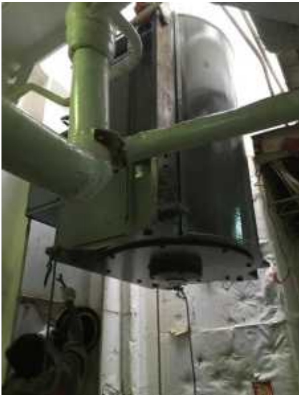
Shaft Generator lifted in vertical position due to insufficient clearance of sky light for entry
