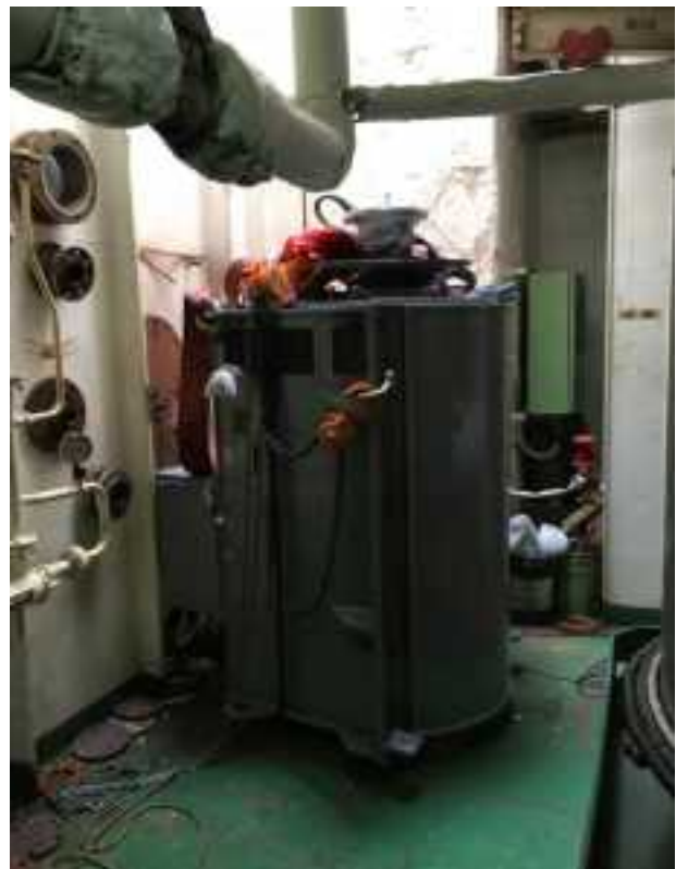
Shaft Generator lifted in vertical position due to insufficient clearance of sky light for entry
