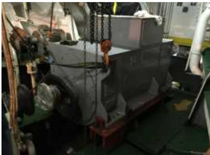
Shaft Generator were shifted into position at 0430hrs
