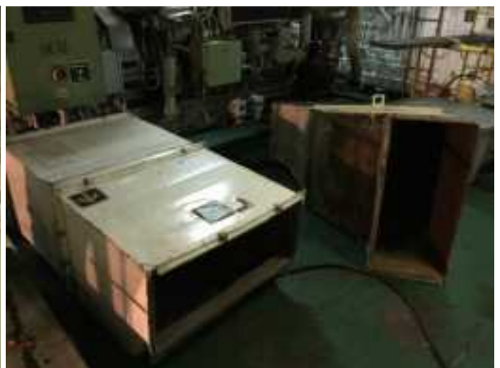
Removal of top level air ducting section to give way to shaft generator
