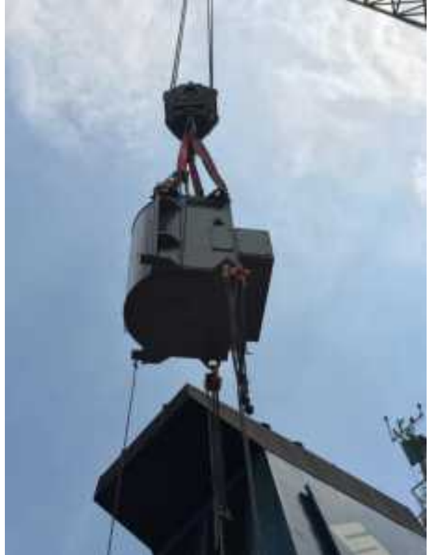
Shaft Generator lifted in vertical position due to insufficient clearance of sky light for entry
