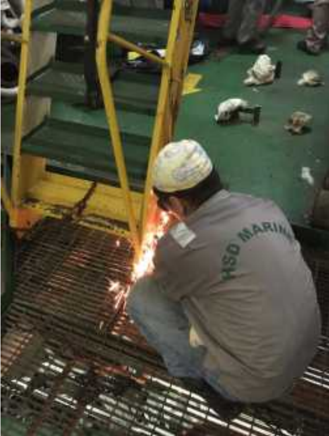
Removal of tween deck's ladder
