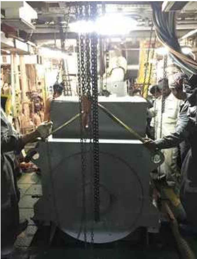
Adjusting alignment of generator & jacking bolts of foundation
