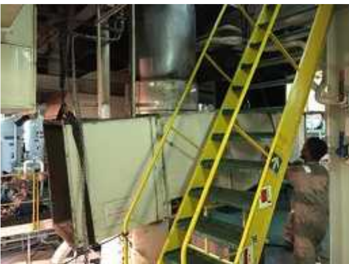
Removal of top level air ducting section to give way to shaft generator
