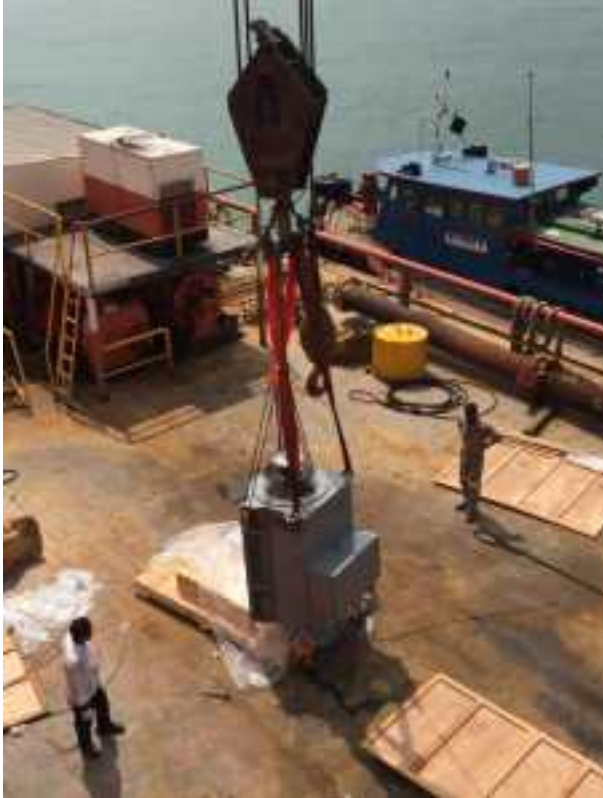
Shaft Generator lifted in vertical position due to insufficient clearance of sky light for entry
