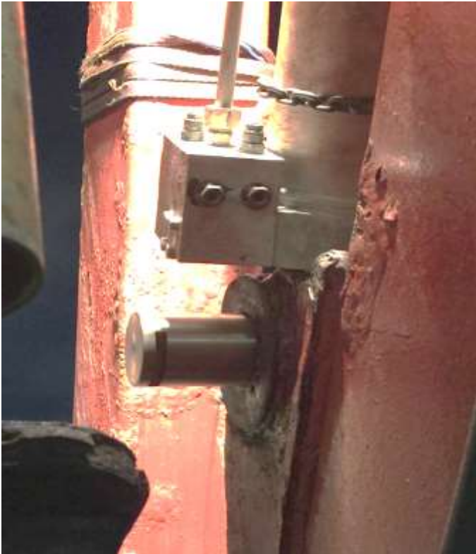
Inserting pins after hydraulic cylinder aligned
