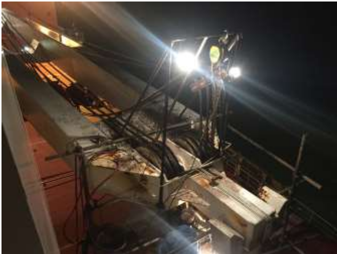
Fabricated lifting frame in situ & installed on top side of crane jib head
