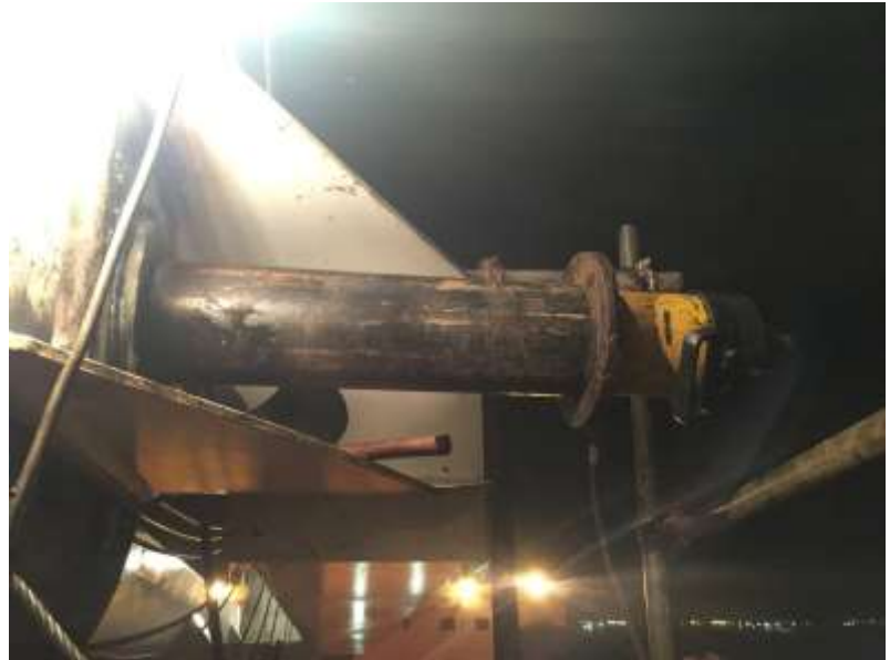
Attempted several times to extract intermediate pin, not successful.
