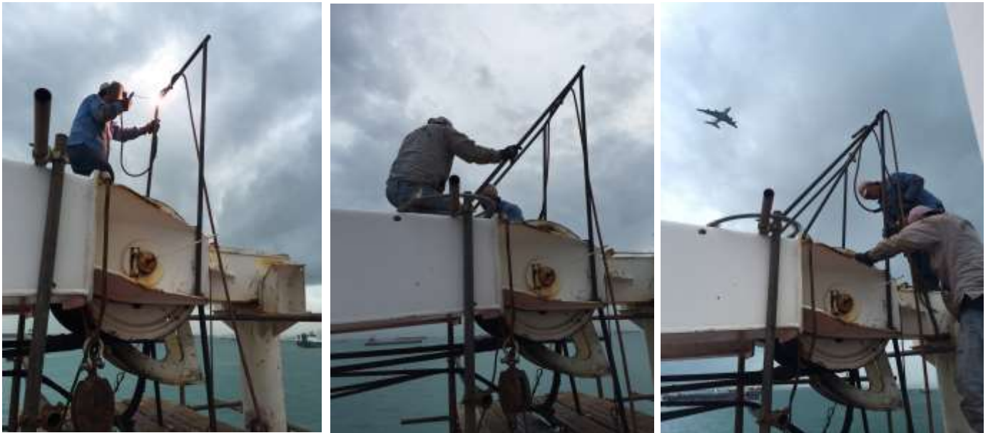
Fabricated lifting frame in situ & installed on top side of crane jib head
