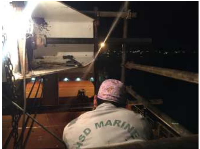
Fabricated lifting frame in situ & installed on top side of crane jib head
