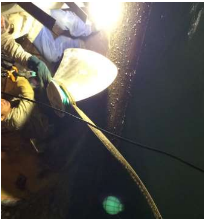
Transferred and installed thruster's blade one by one, applied grease on O rings and reassembled bolts connections,
