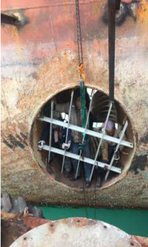
Reinstall back the guard grip
