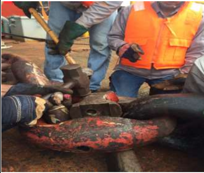
Connecting Of Kentre Shackle from Anchor Chain To Anchor Swivel
