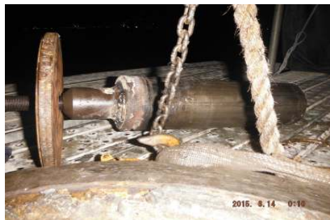
Continued extraction with hydraulic tools at 1000BAR pressure threaded stud broken and nut cracked fall off after Keep trying extraction the Sheave Pin were out.
