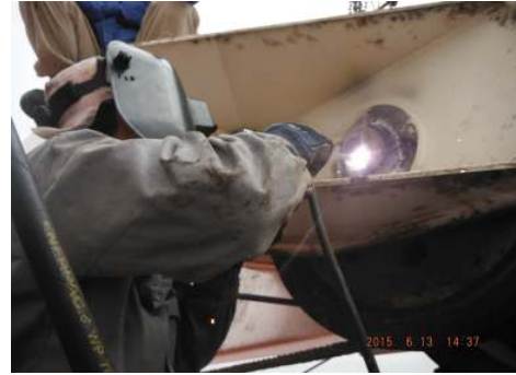
New nut were welded
