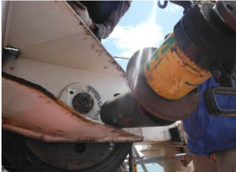
During the extraction nut were cracked and fall off
