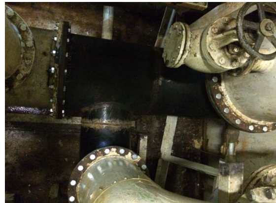
Upon completion carried out rubber coating in both pipes.
