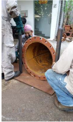
Reducer pipe were templated
