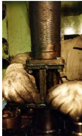
Cleaned the fuel oil pipes with diesel oil and installed and new gasket were changed
