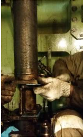
Cleaned the fuel oil pipes with diesel oil and installed and new gasket were changed
