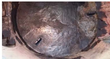
Applied one layer primer coating and mixed rubber elements in situ
