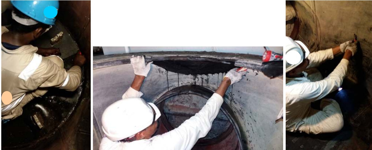
Cropped off all the damaged rubber coating in the sea chest.
