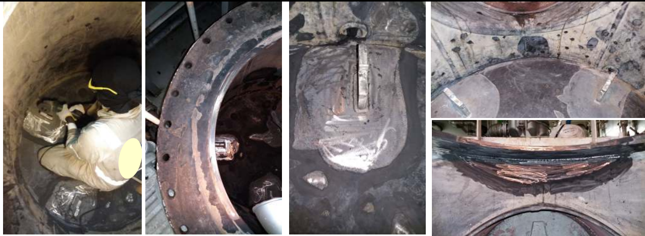
Well grinded all the spots and made smooth surface.
