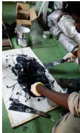
Applied one layer primer coating and mixed rubber elements in situ
