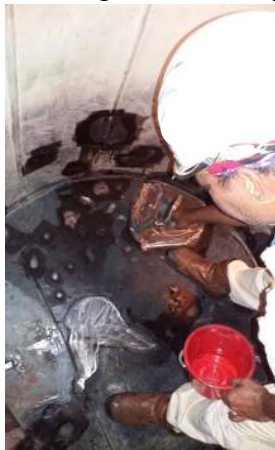
Applied one layer primer coating and mixed rubber elements in situ
