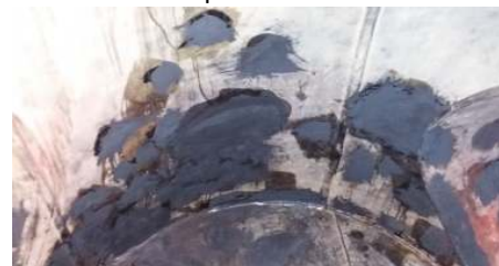
Applied New Rubber coating on all the spots
