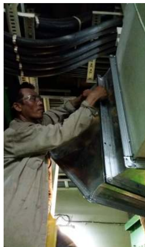
All Elbows Joints and End Caps were fitted accordingly and Silicone paste were applied in all the joint corners.
