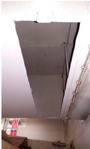
Measured and crop off the existing ducting in order to do the modification.
