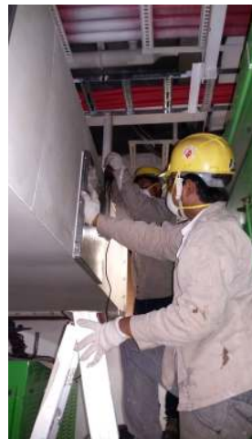
All Elbows Joints and End Caps were fitted accordingly and Silicone paste were applied in all the joint corners.
