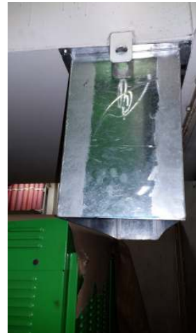
All Elbows Joints and End Caps were fitted accordingly and Silicone paste were applied in all the joint corners.
