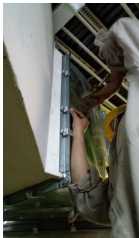
All Elbows Joints and End Caps were fitted accordingly and Silicone paste were applied in all the joint corners.
