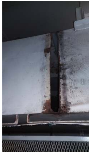
Measured and crop off the existing ducting in order to do the modification.
