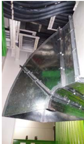
All Elbows Joints and End Caps were fitted accordingly and Silicone paste were applied in all the joint corners.
