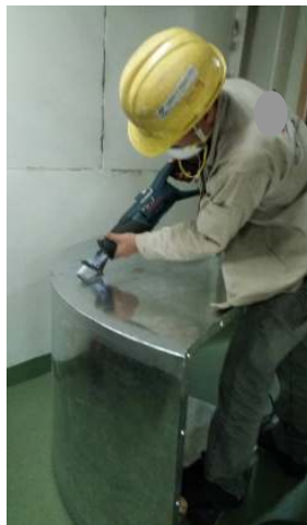
Elbows and End Caps modification, Filter renewal, and Insulation were carried out in situ.
