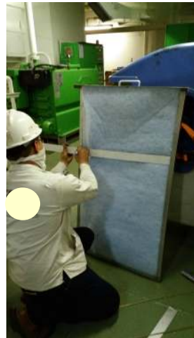
Elbows and End Caps modification, Filter renewal, and Insulation were carried out in situ.
