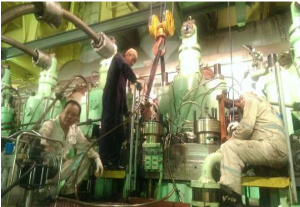
Hydraulic tool was installed and tighten the Cylinder head nut
