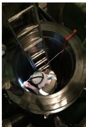
Reconditioned liner was installed with new O ring and calibrated
