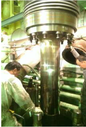
Piston was mounted back and changed new gasket
