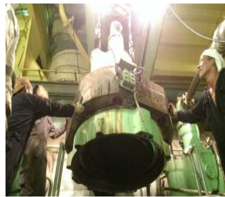
Removed all the connections. Hydraulic tool was installed and loosen the nut and cylinder head dismantled.
