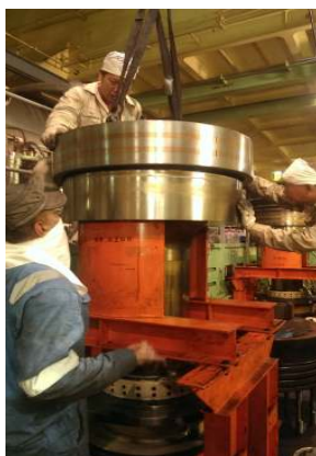
New piston skirt installed
