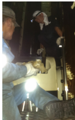
Dismantled lock bolts
