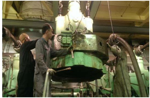
Cylinder head back in placed
