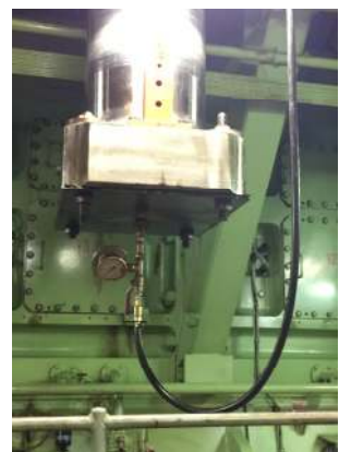
Pressure test performed No leaking was found
