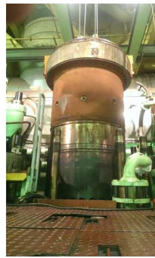
Liner pulled out
