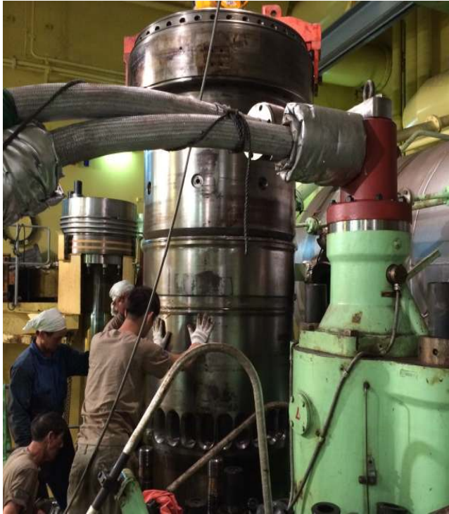
Install the spare piston and liner
