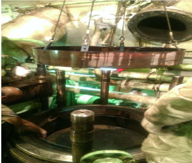
Remove fire ring and piston stuffing box mounting bolt
