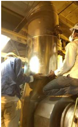
Fabricated generator exhaust bellow covers were installed and tightened with screws
