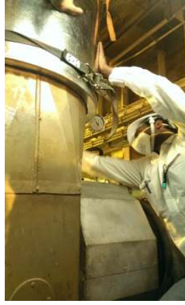
Fabricated generator exhaust bellow covers were installed and tightened with screws
