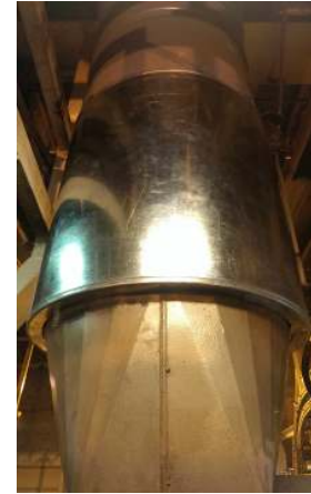
Fabricated generator exhaust bellow covers were installed and tightened with screws
