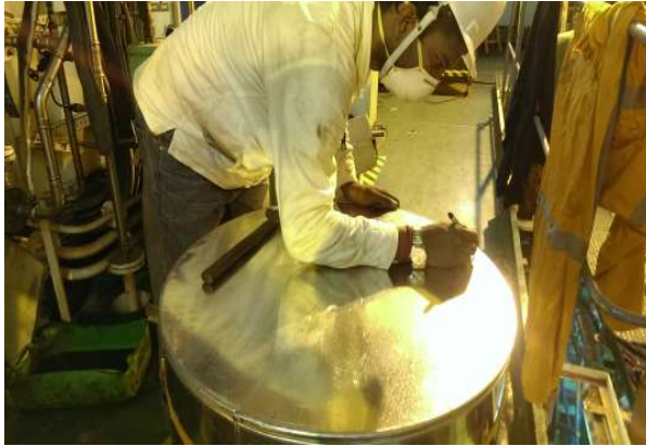
Covers for generator exhaust bellows were measured and fabricated in situ
