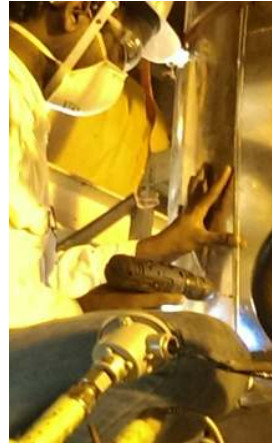
Fabricated generator exhaust bellow covers were installed and tightened with screws
