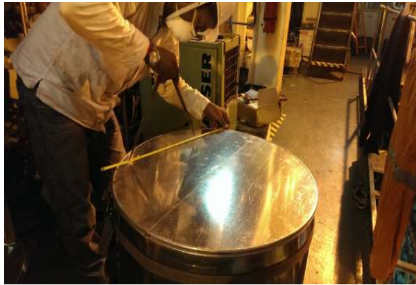
Covers for generator exhaust bellows were measured and fabricated in situ
