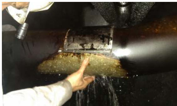
Clamped up and tightened
